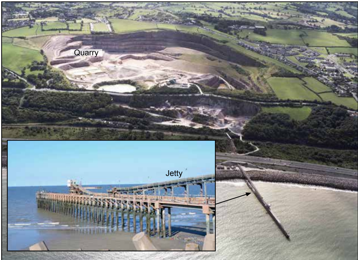
Figure 1: Raynes quarry and Jetty
