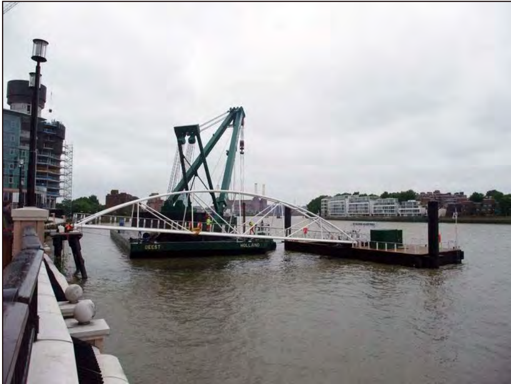
Figure 3: Installation of the pier linkspan at St George Wharf
