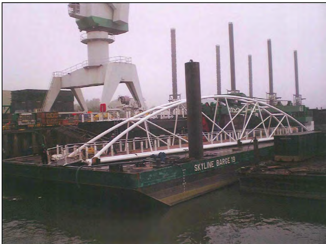
Figure 1: Skyline Barge 19 with the pier linkspan secured on deck
