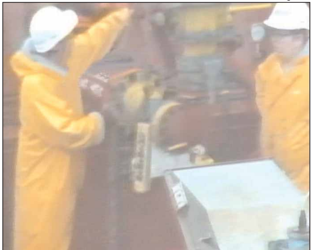
Two shore operators connecting the loading arm to ship's manifold
