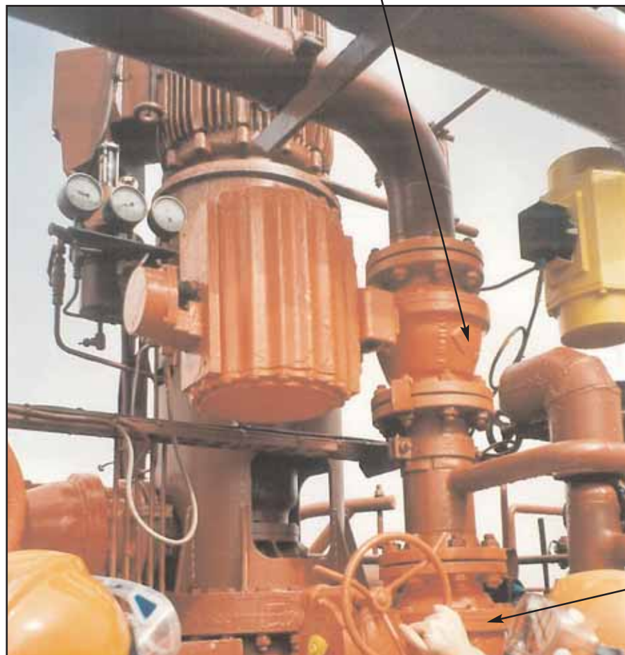
Forward tank loading valves
