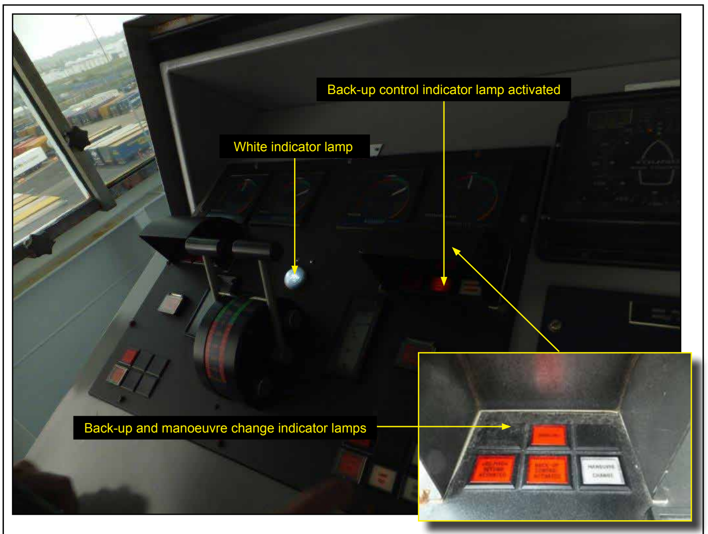
Figure 4: Comparative brightness of bridge wing console indicator lights
