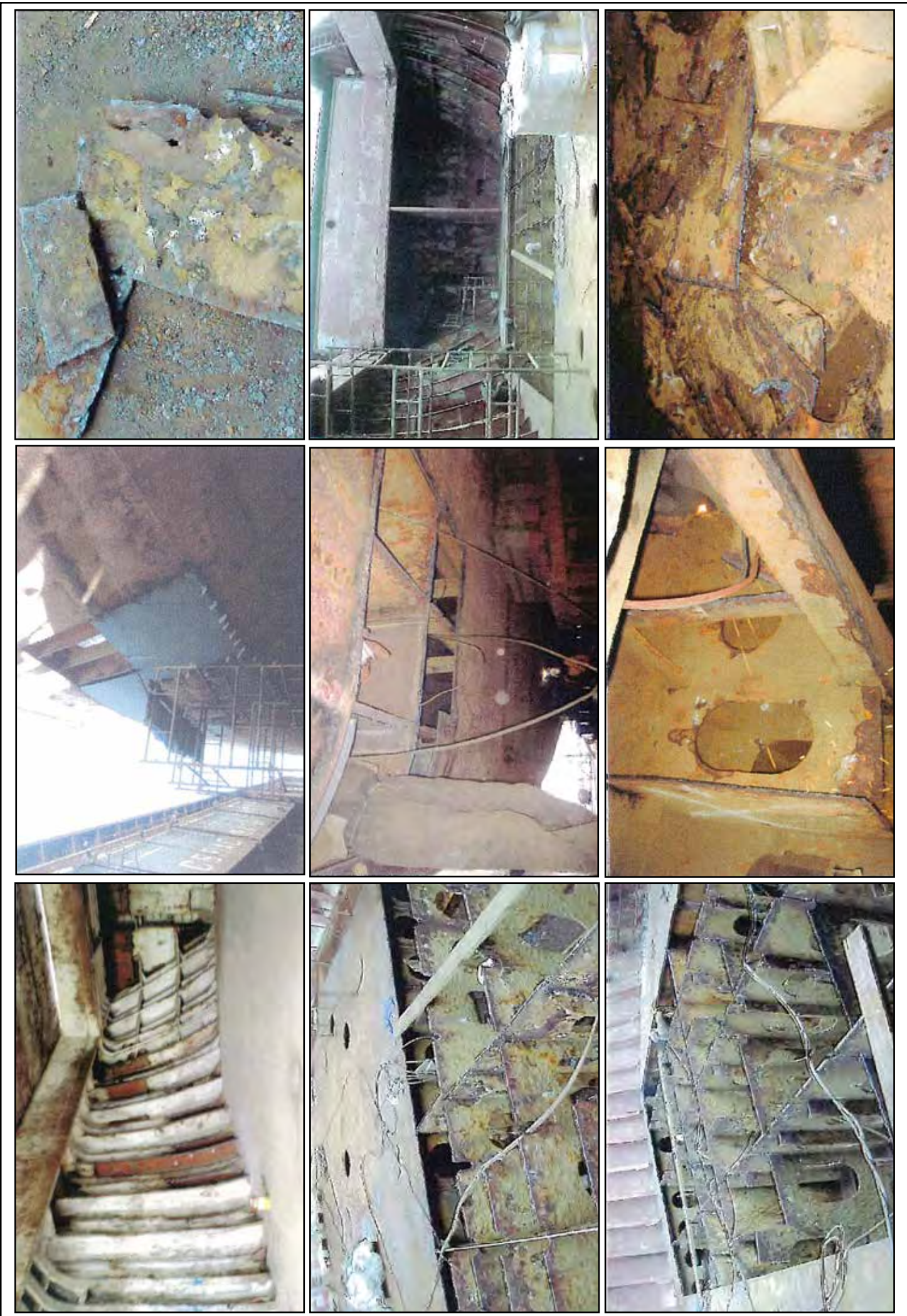
Figure 40: Repair work underway in Liepaja in 2006
