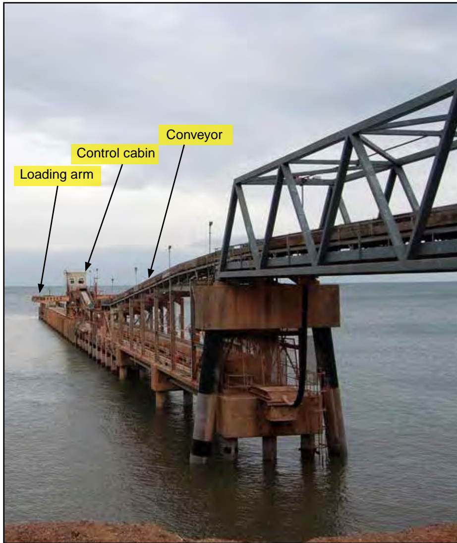
Figure 50: Raynes Jetty, Llanddulas
