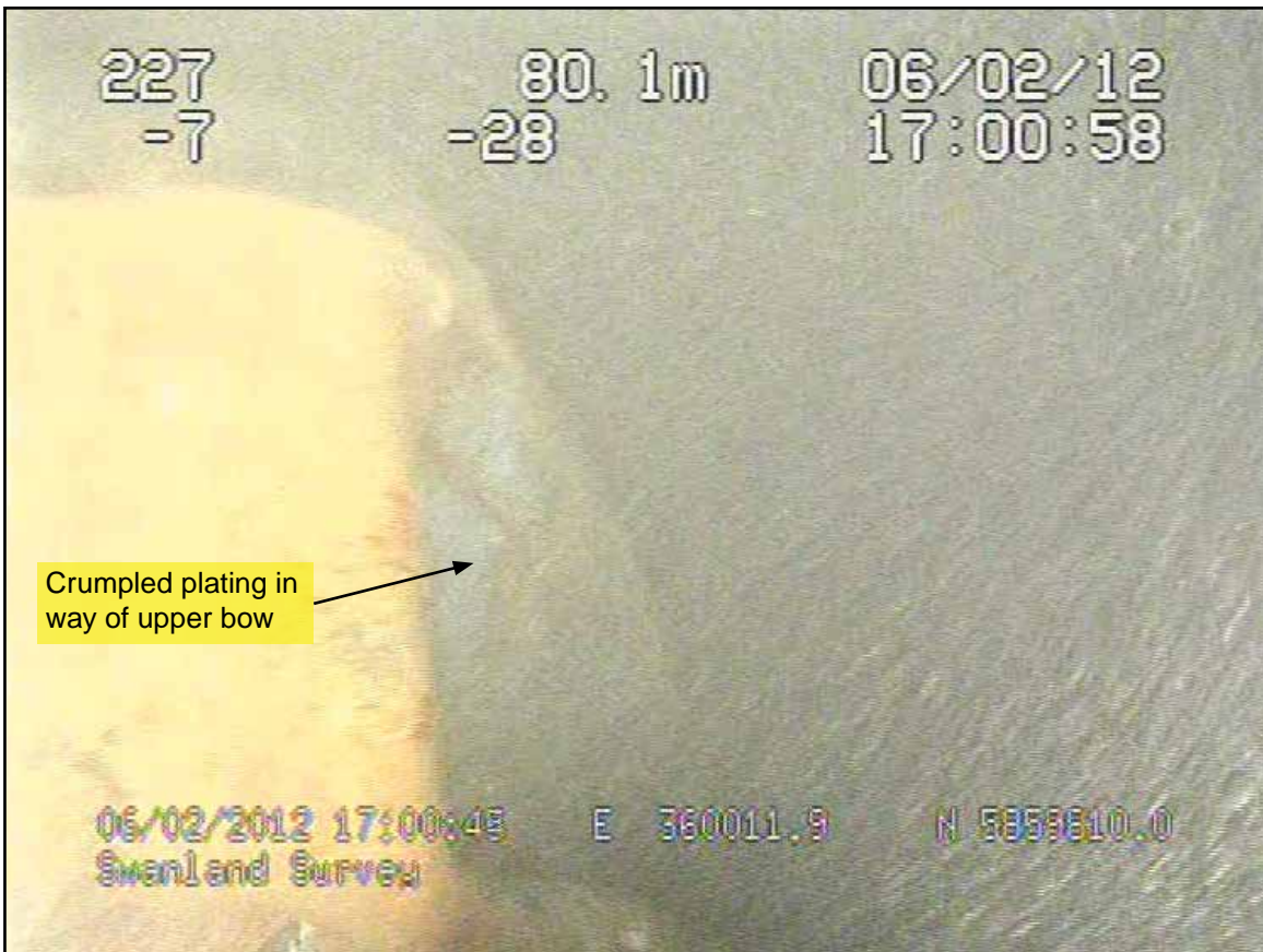
Figures 30a and 30b: Stills from ROV footage showing crumpling of the top of the stem and bulwarks
