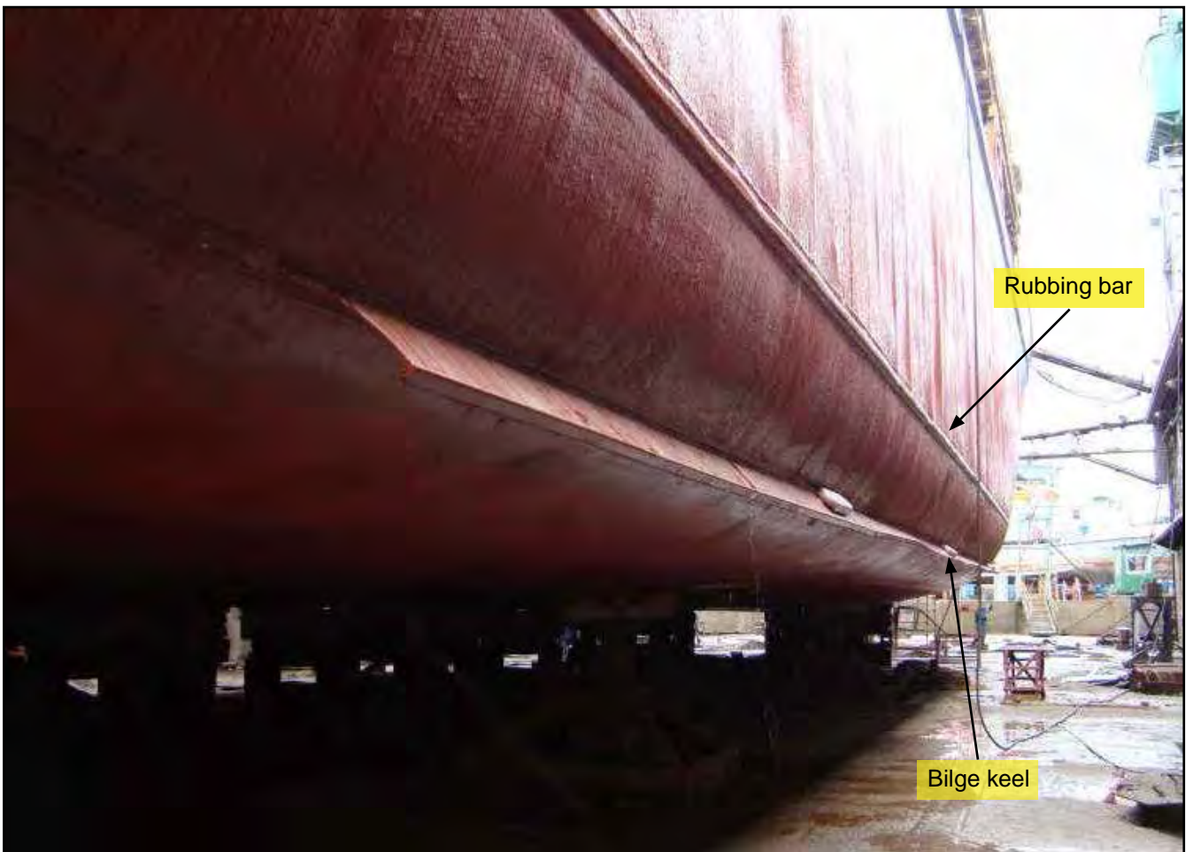
Figures 19a and 19b: Swanland in 2002 showing location of rubbing bar above bilge keel
