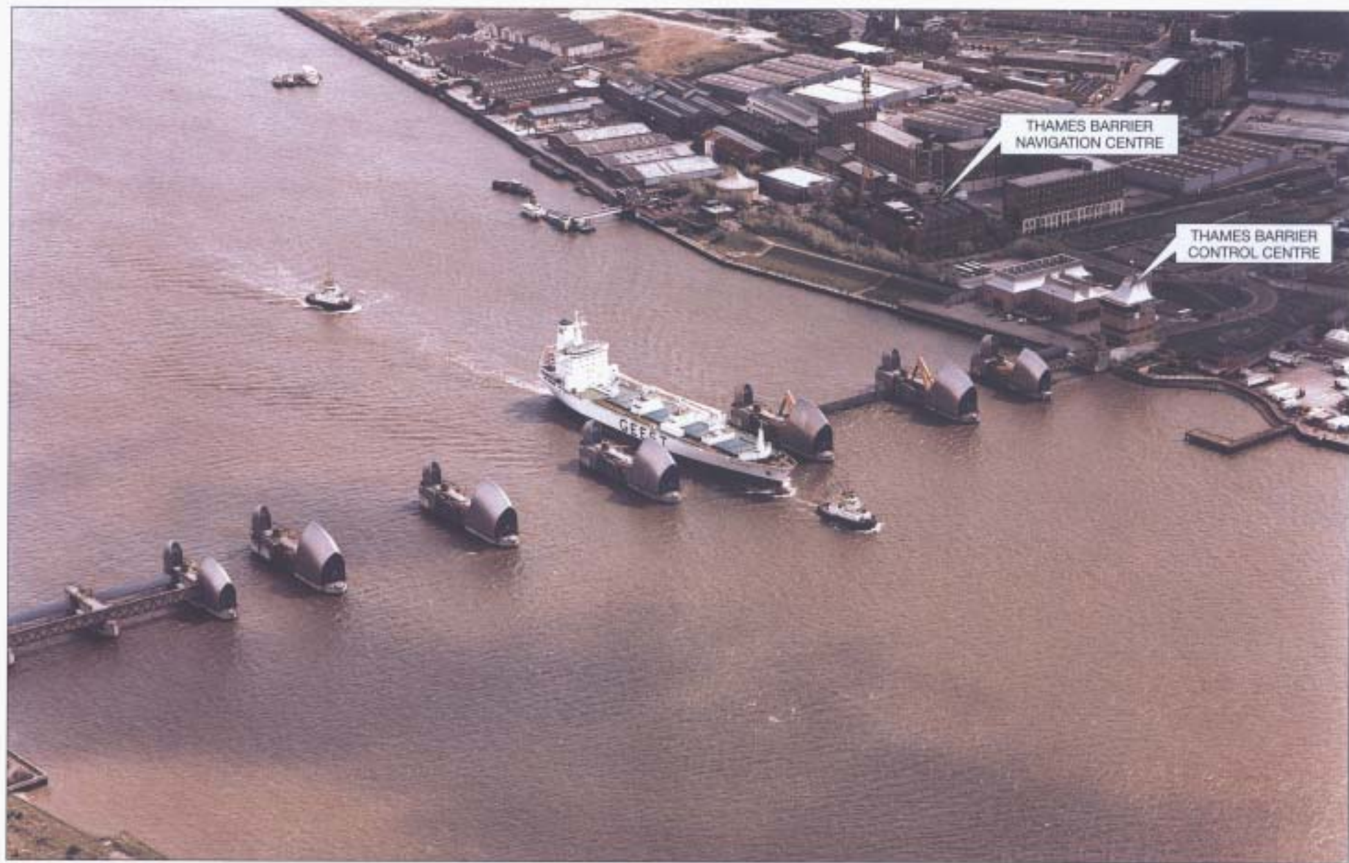
Figure 2: The Thames Barrier [photograph courtesy of Chorley & Handford Limited]
