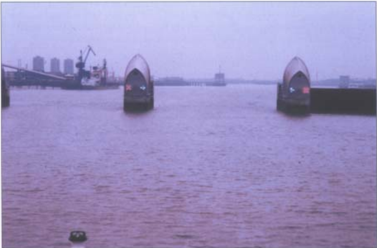
Figure 9: Navigation lights (span open)
