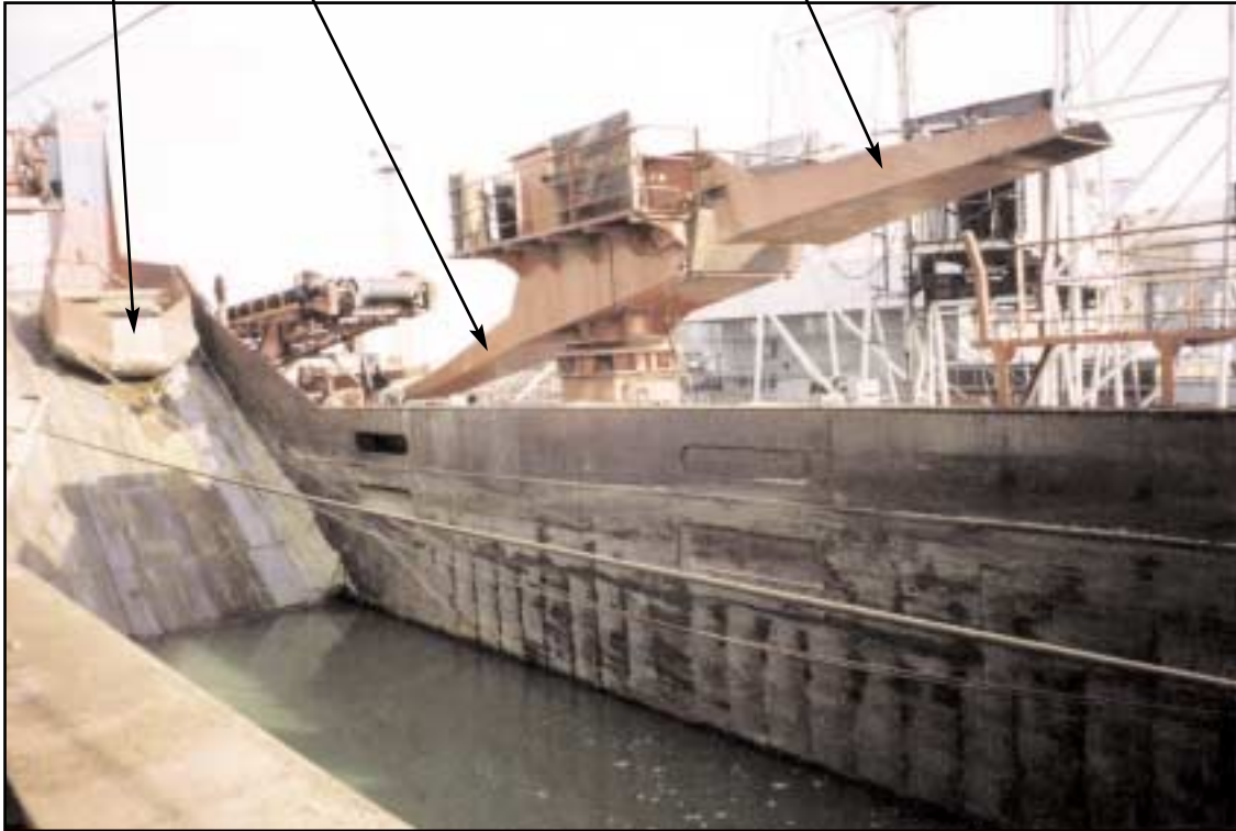
View across cargo hopper of port bucket arrangement and aft loading tower
