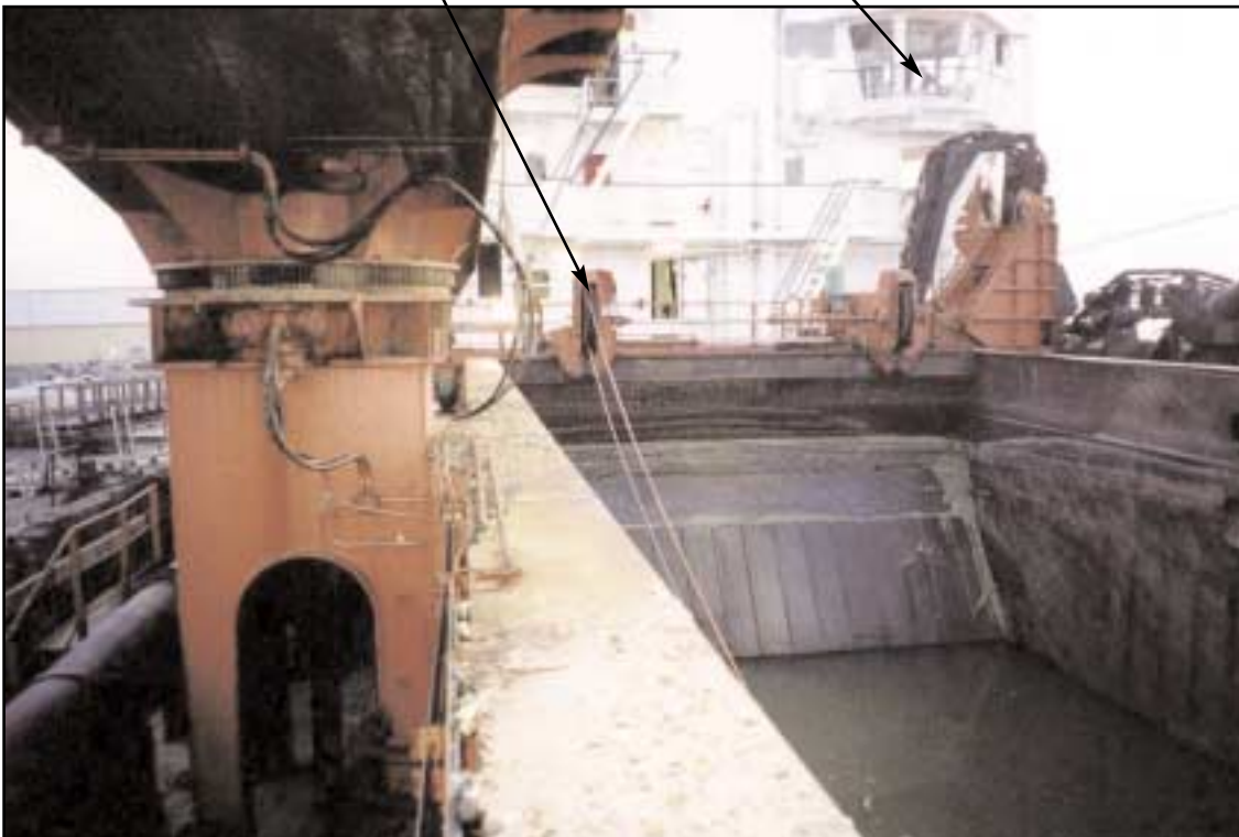
View of sheaves at forward end of hold, from aft loading tower
