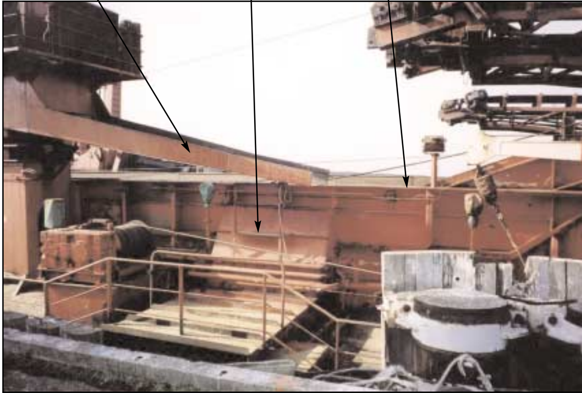
View of aft tower reject chute and platform
