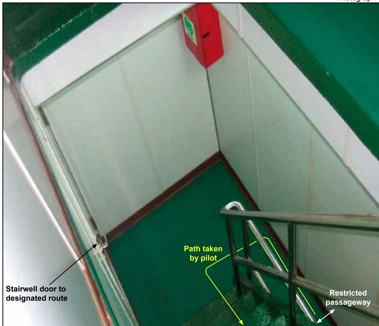
Internal stairs within Leonis
