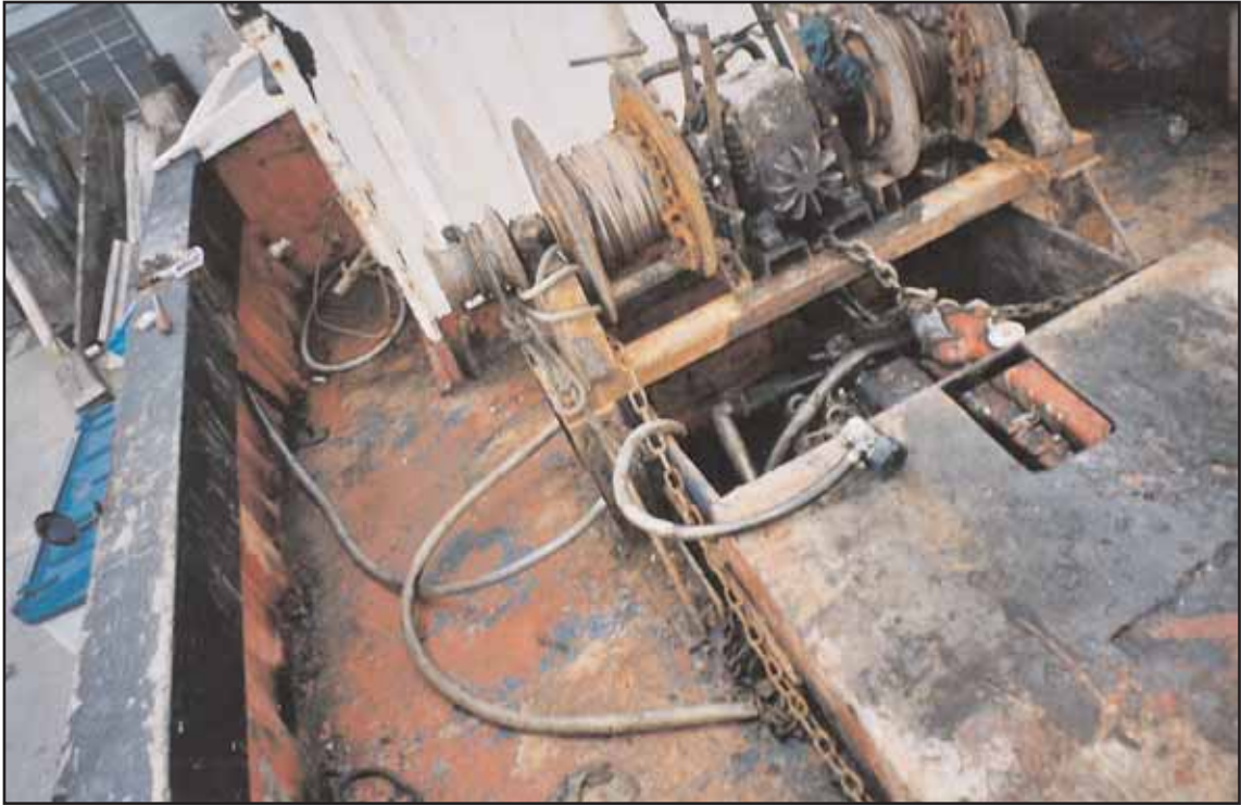
Engine hatch and coaming penetrations
