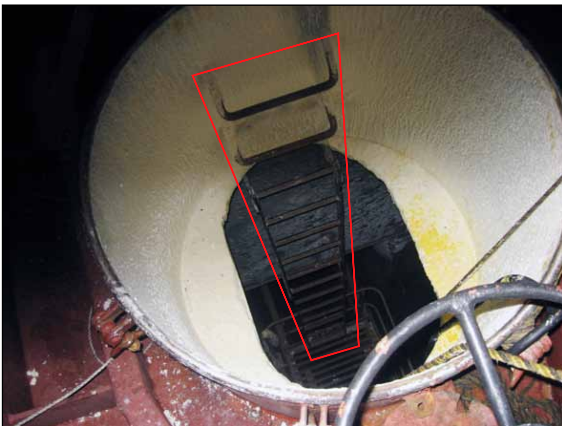
No 2 cargo tank - vertical ladder
