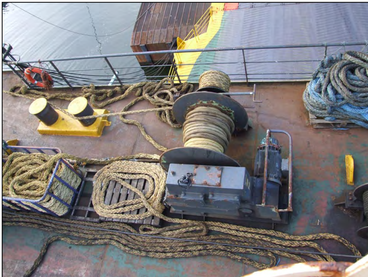
Stern line electric mooring winch
