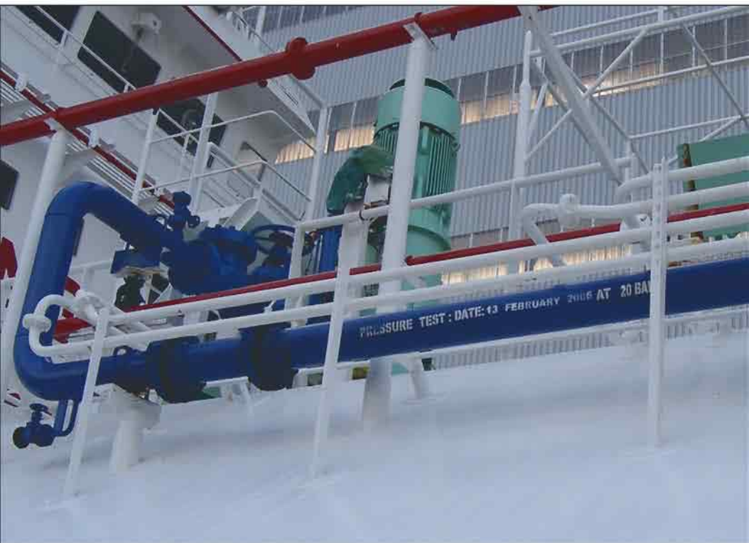
Pipework pressure test
