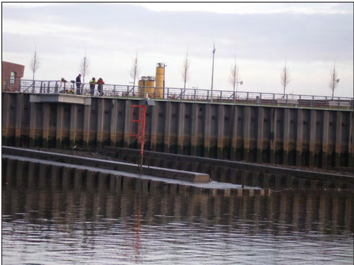
Hazard and navigation mark
