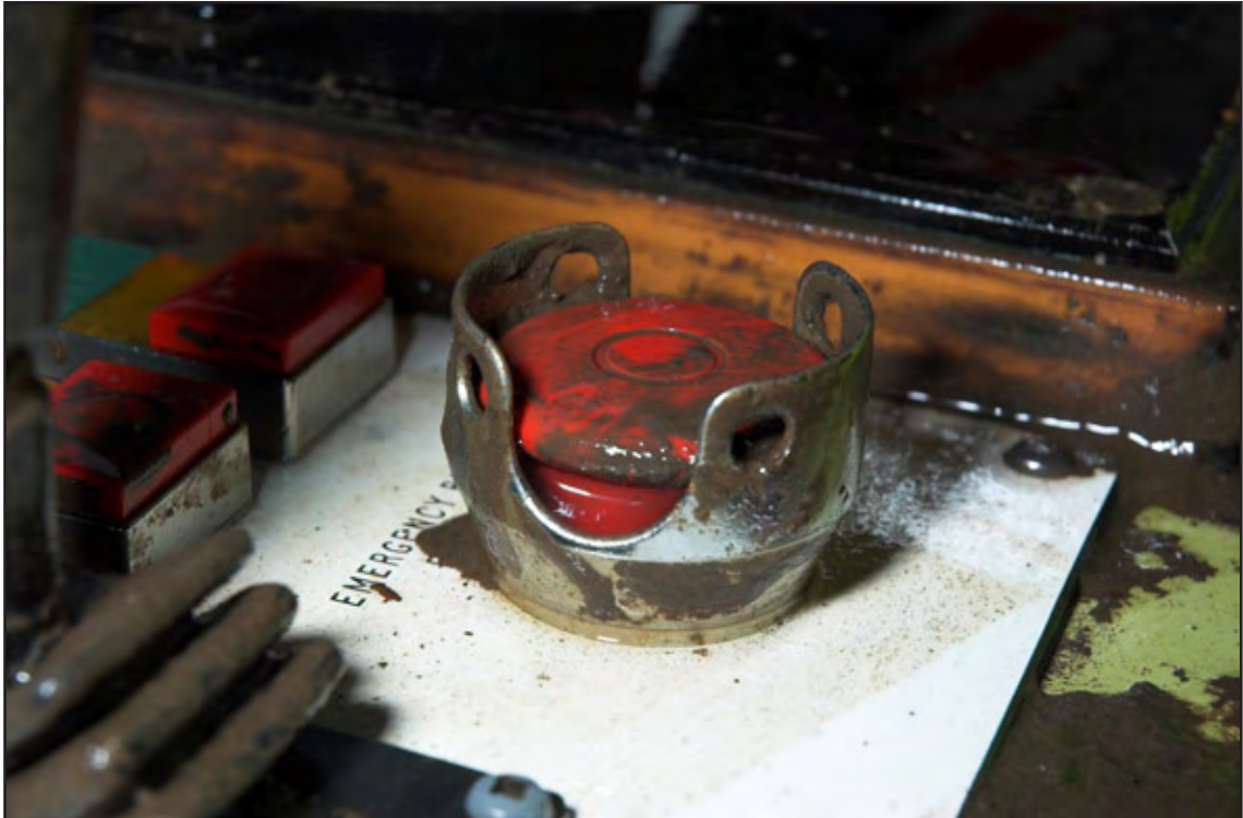
Starboard emergency release button
