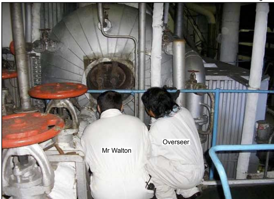
Re-enactment of Mr Walton's and the overseer's positions in front of the starboard boiler steam drum immediately prior to the explosion
