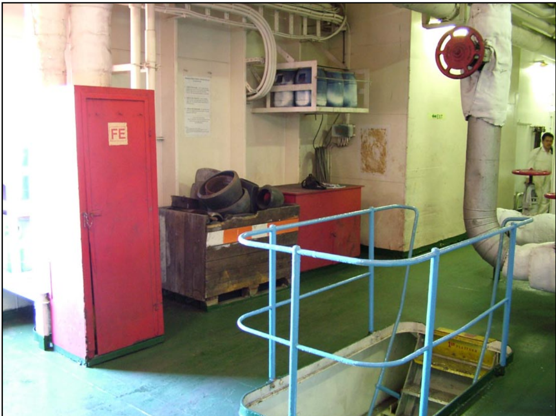
After view of the starboard boiler steam drum top plate level
