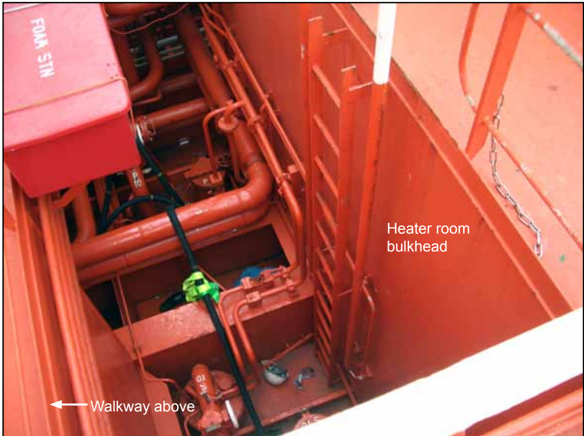
Walkway aft of P10 inboard Butterworth hatch
