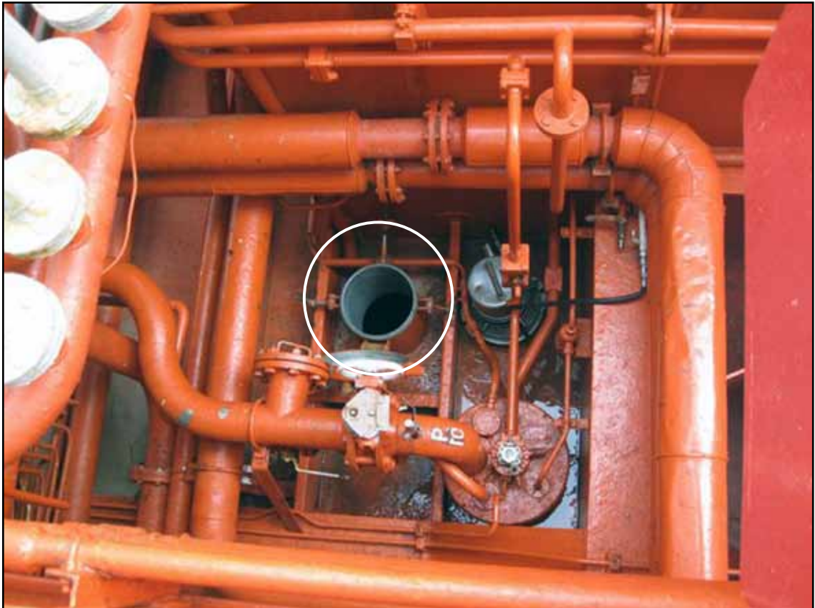
Cargo tank P10 open inboard Butterworth hatch
