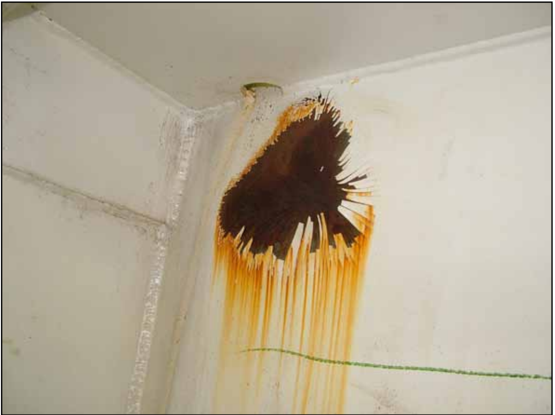
Hull indentations - port side bow thruster room
