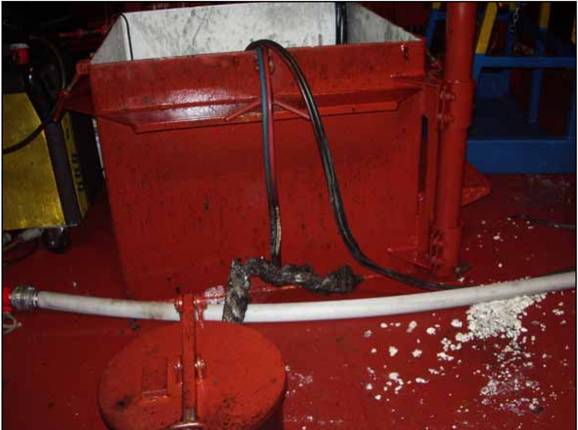
Acetylene and oxygen hose fire damage
