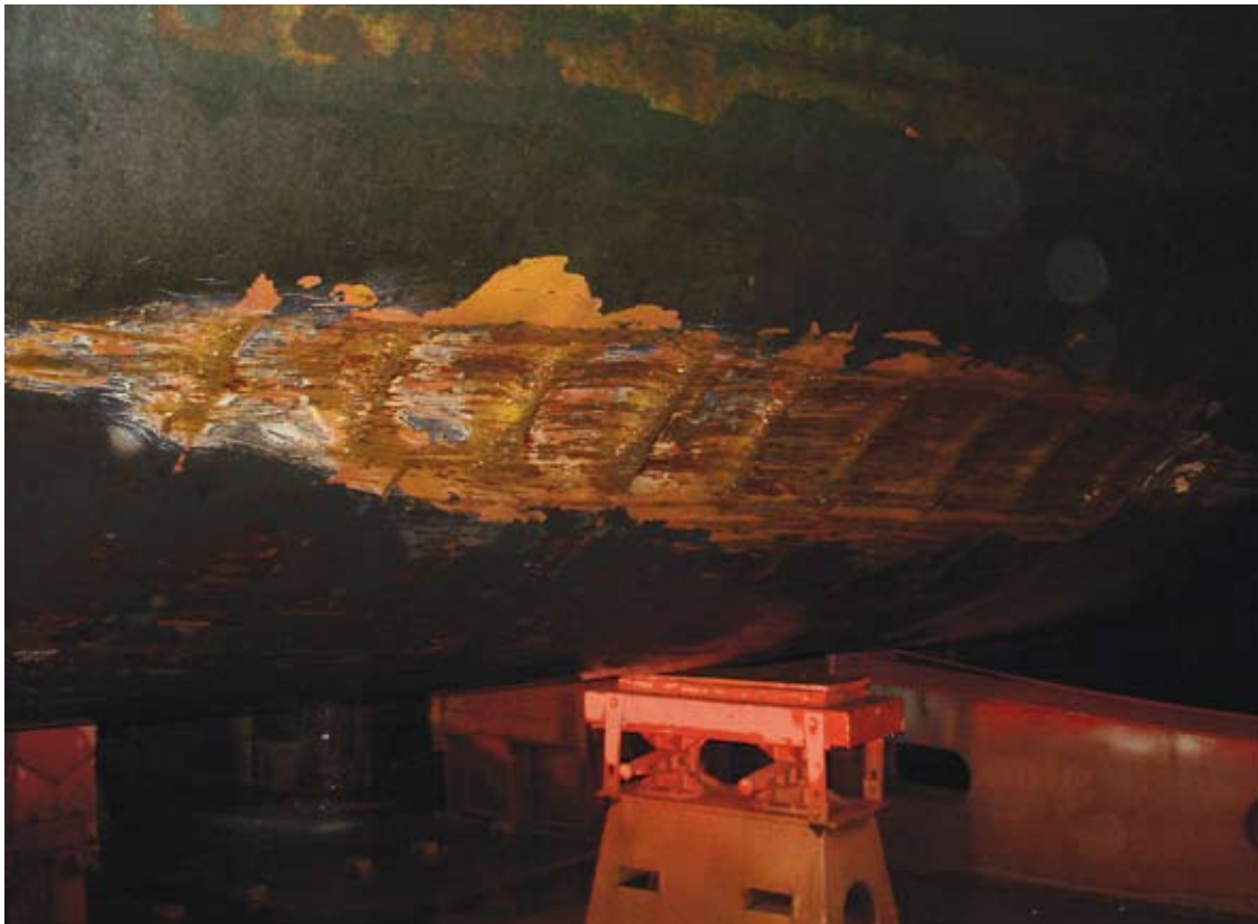
Damage below the waterline
