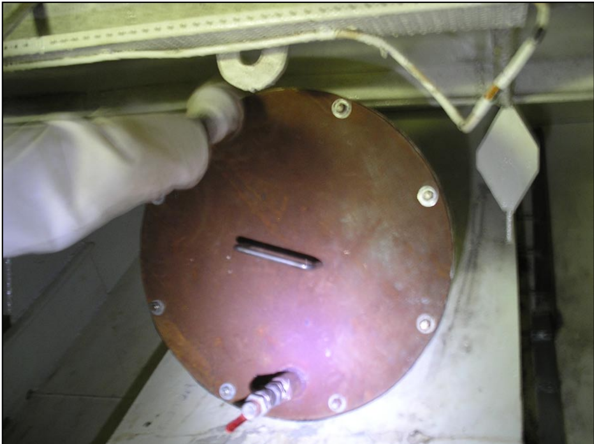
Closing of ventilation duct
