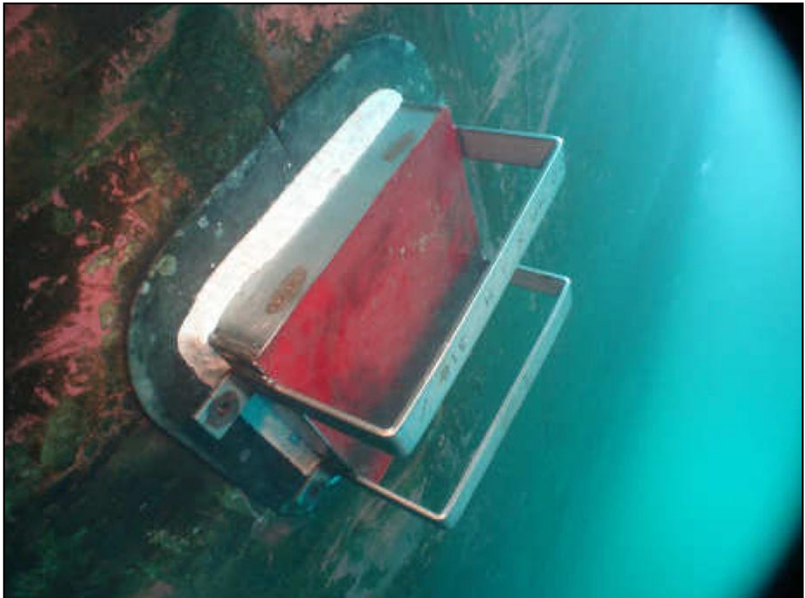
Temporary repair to No.2 deep ballast tank
