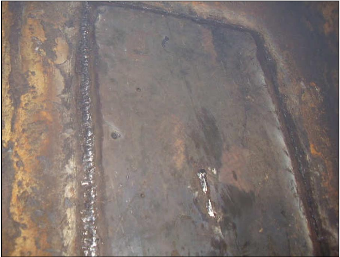
Temporary repair to the forepeak
