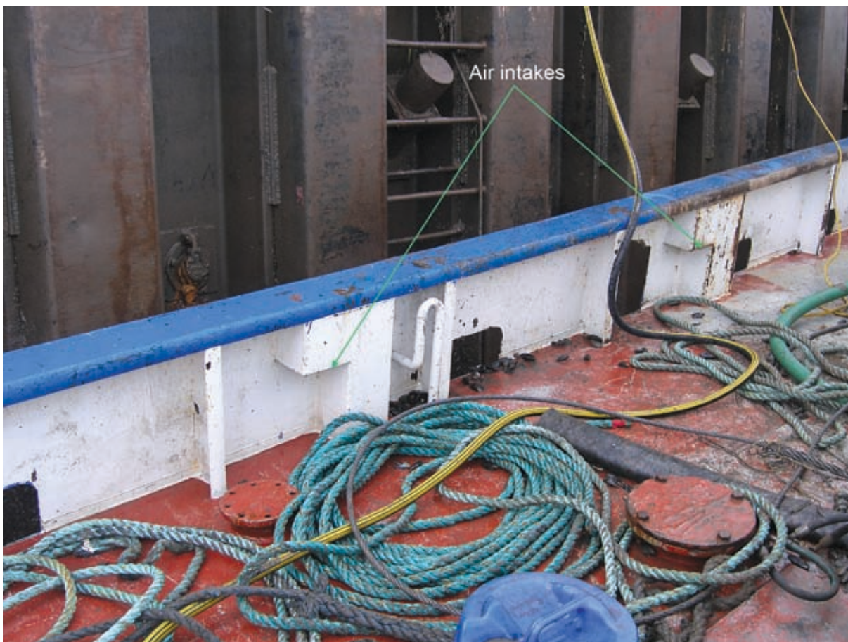
Figure 1: Deck, showing engine room air intakes
