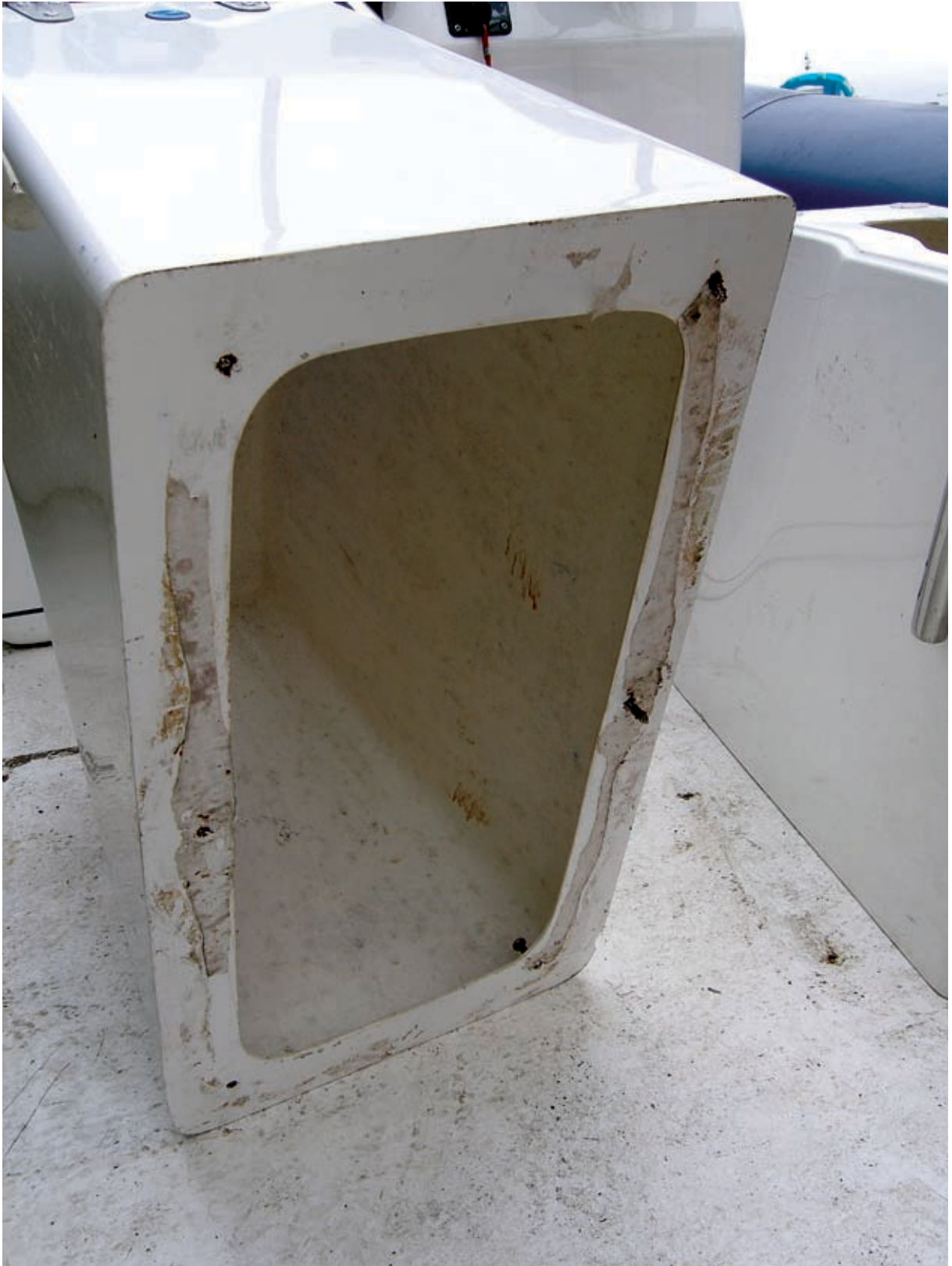
Vessel's seat note: wide spacing of securing screws and poor coverage of sealant
