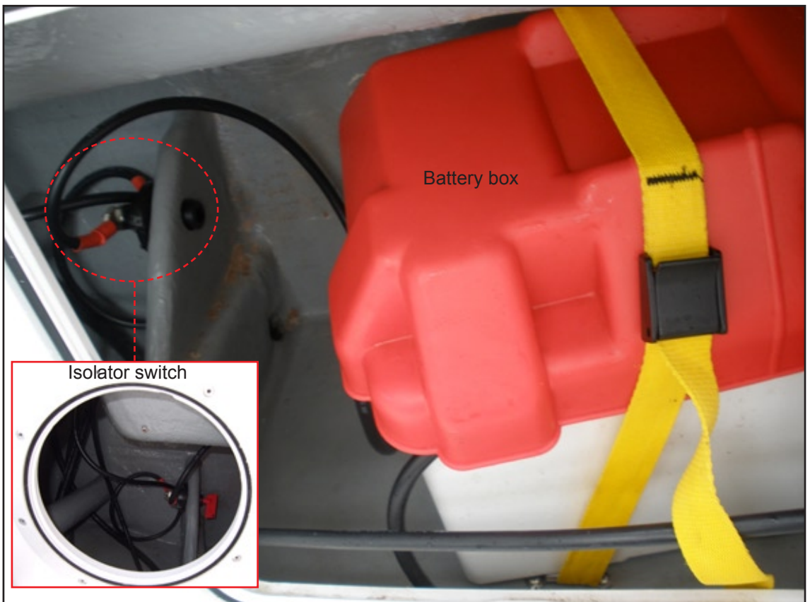
Partner 1 battery box and electrical isolator switch
