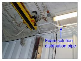
The debris found in the nozzles and piping is most likely to have been rust and scale that had built up in sections of pipe in which water and/or foam solution had previously been trapped. This debris would then have been distributed along the pipes and into the nozzles during the annual blow through tests and when the system was operated. The resulting blockages were sufficient to prevent the aspiration of the foam solution.
