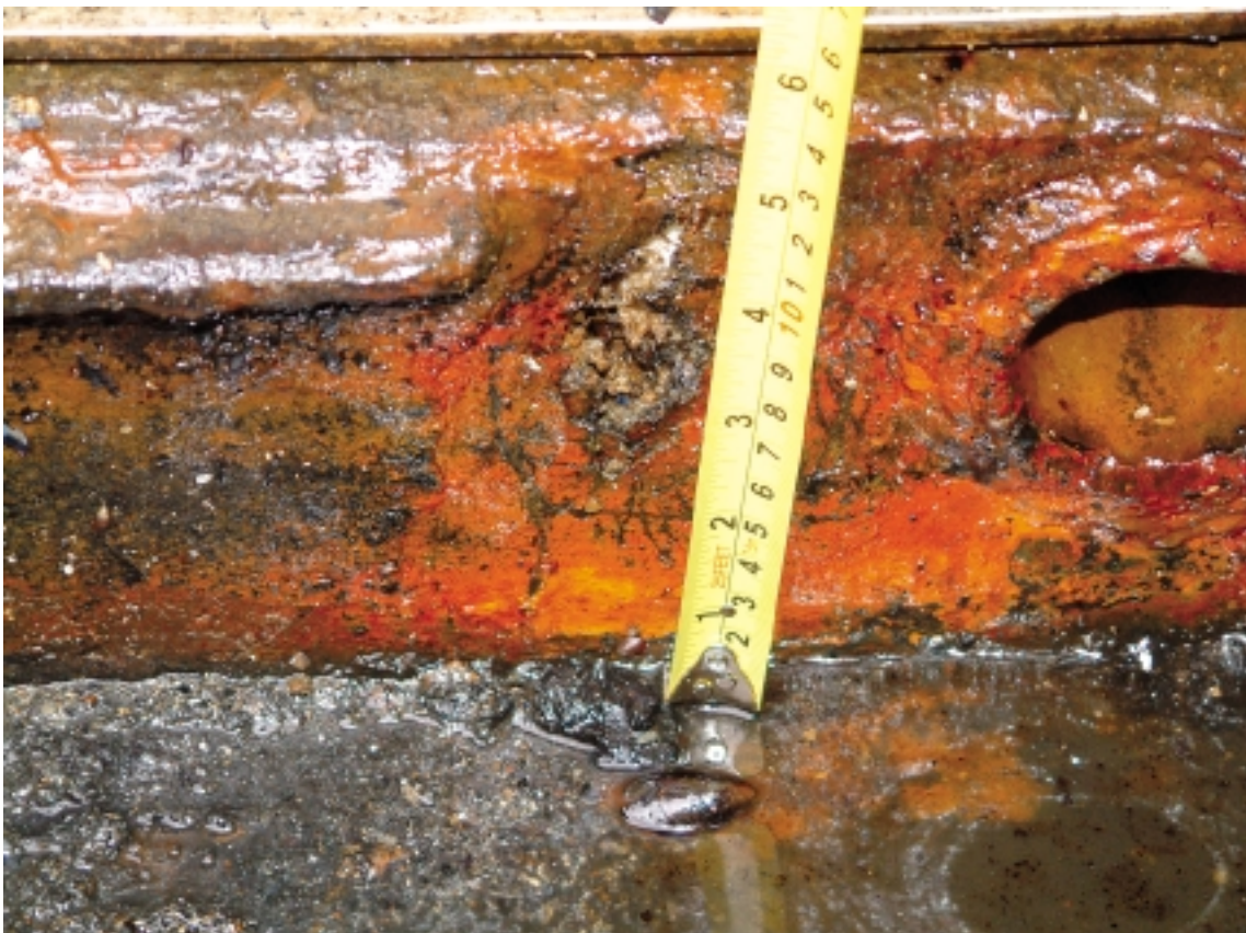
Figure 4 – Plate corrosion
