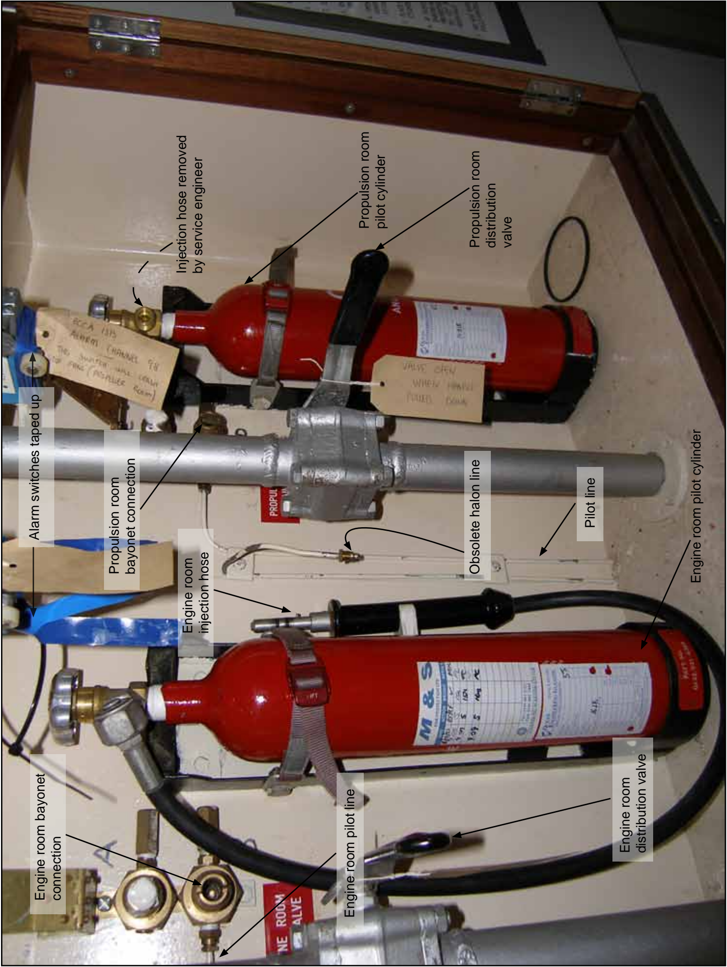
Figure 3: CO 2 control station
