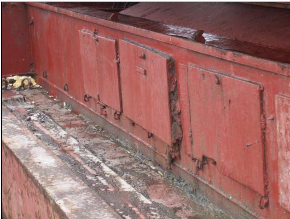
Aft cargo ventilation flaps within hold
