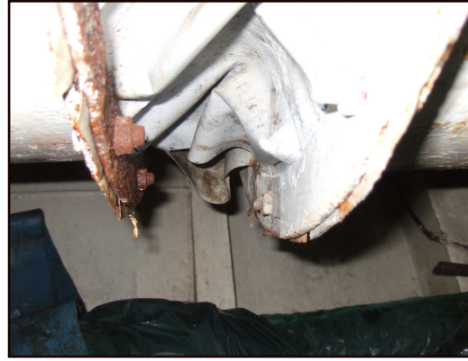
Cut ventilation duct
