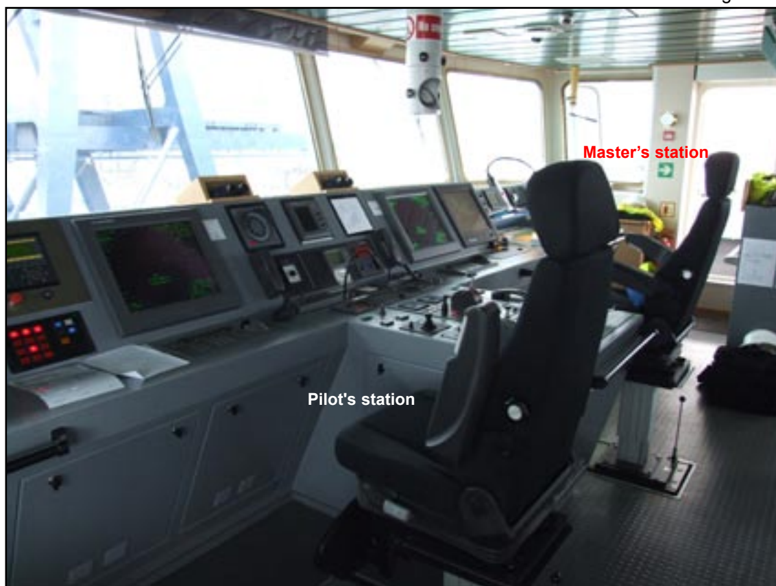
Samskip Courier's bridge showing pilot and master's stations
