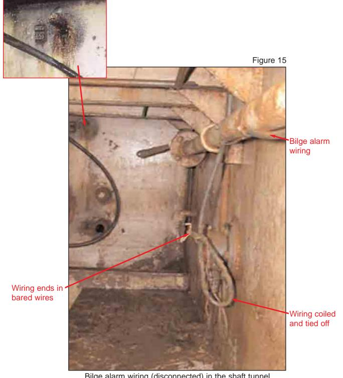
Bilge alarm wiring (disconnected) in the shaft tunnel
