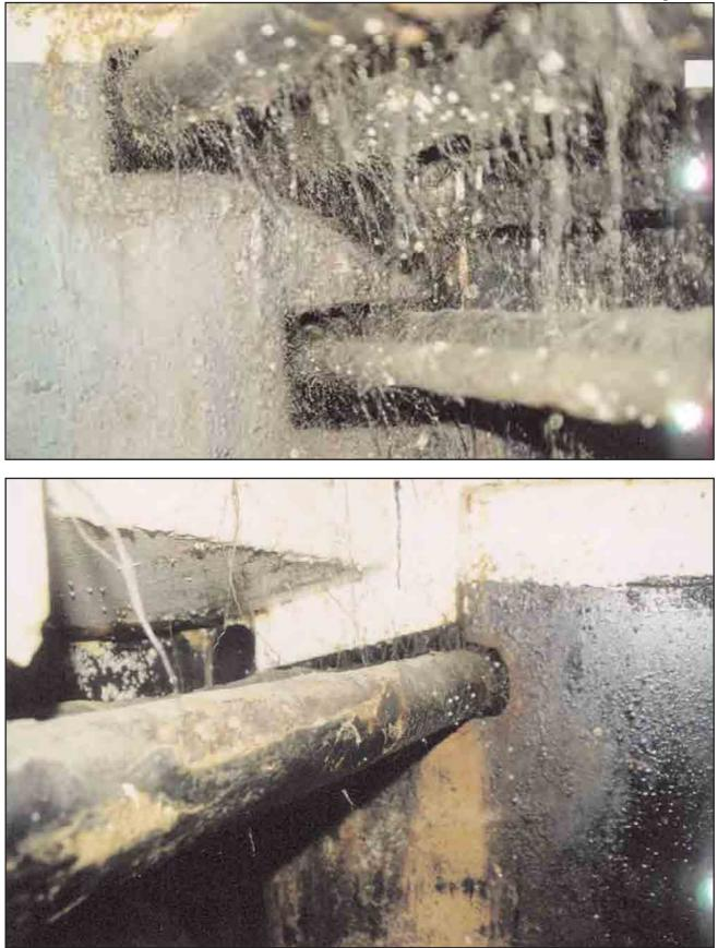
The "watertight" bulkheads showing gaps around pipe penetrations
