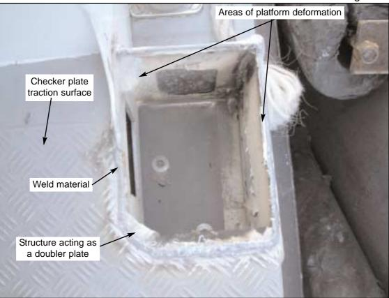
Passenger access platform - structural arrangement
