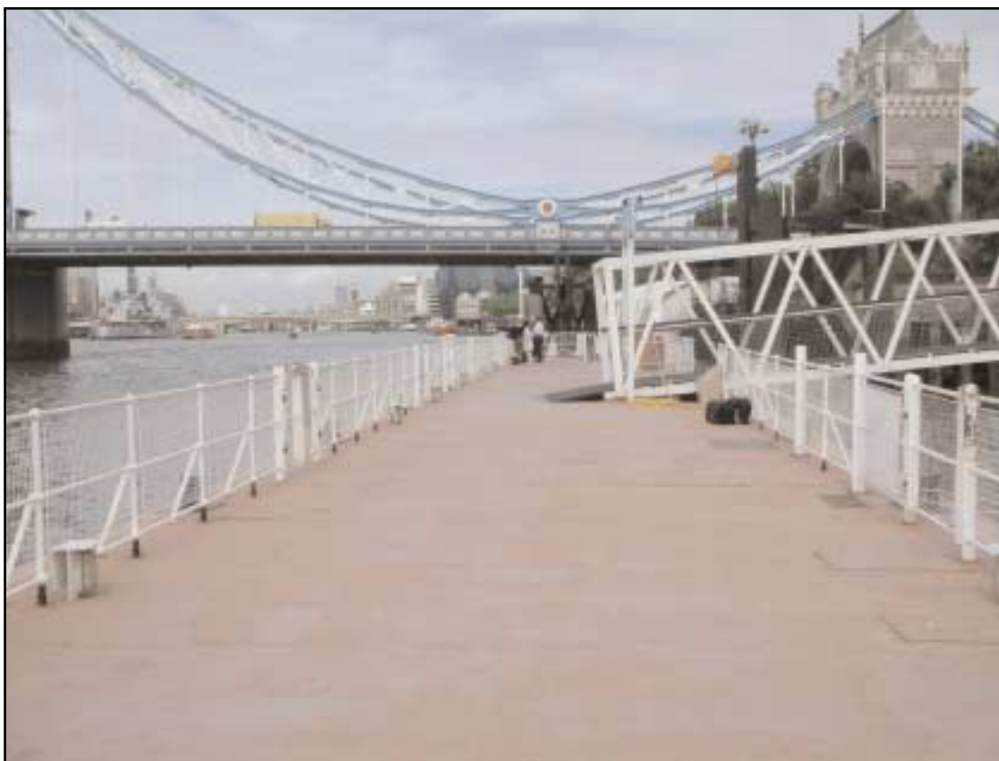
View of Tower Bridge north bank shore arch
