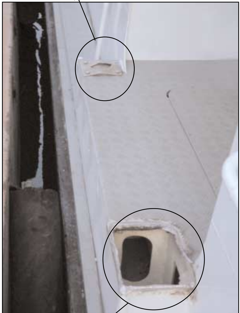
Position of displaced bollard
