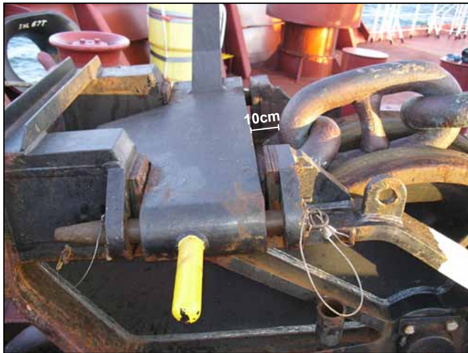
Gap between chain link and stopper
