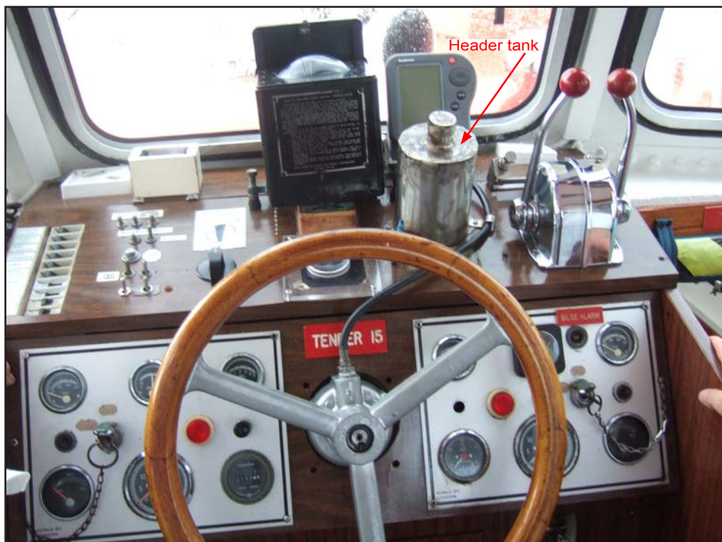
Controls, Tender 15 - with oil header tank fitted
