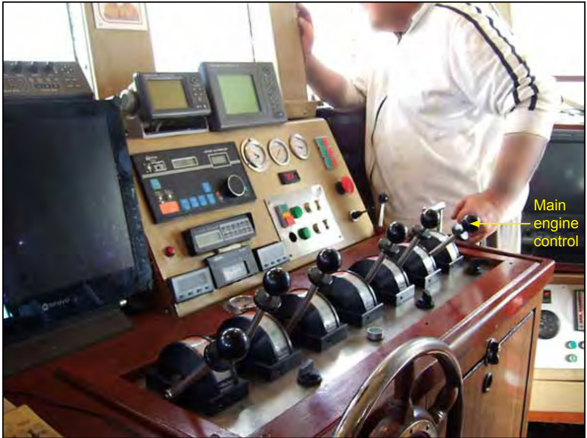
Winch controls for operating fishing gear
