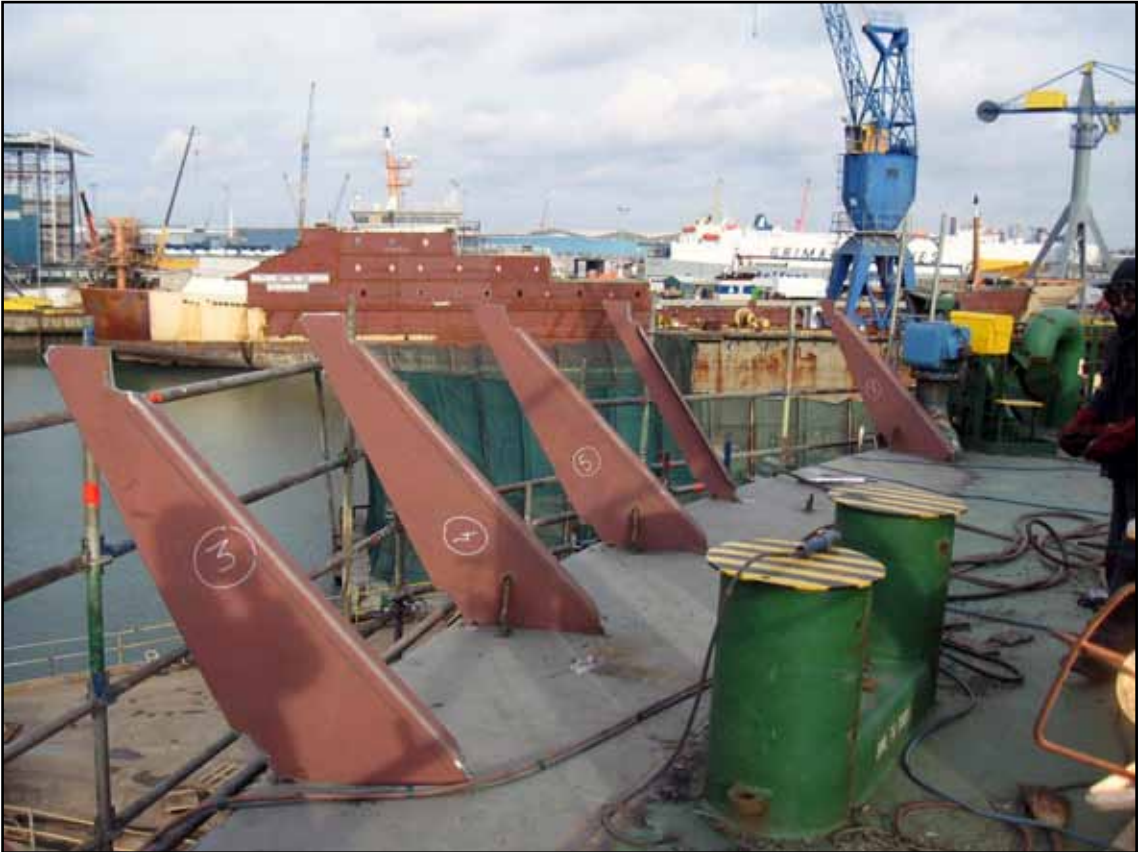
Vallermosa undergoing repairs in Flushing
