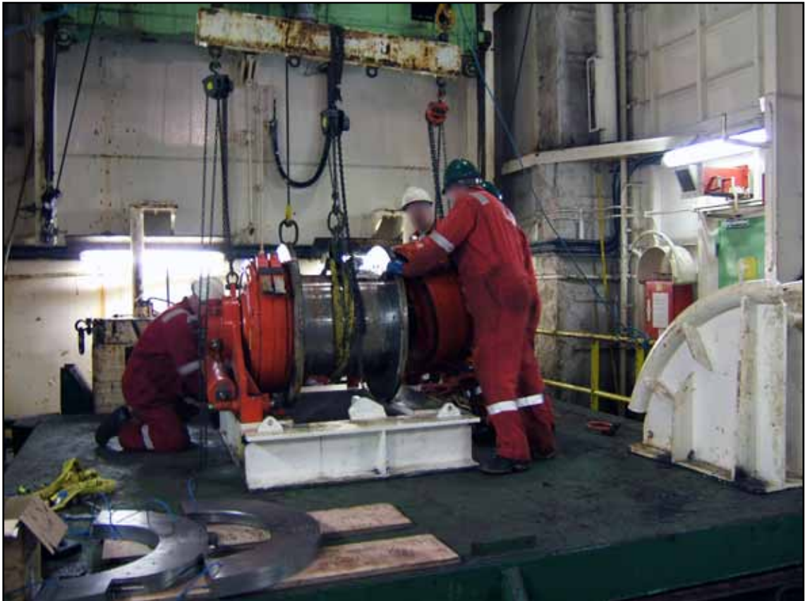
Winch being assembled in bell hanger
