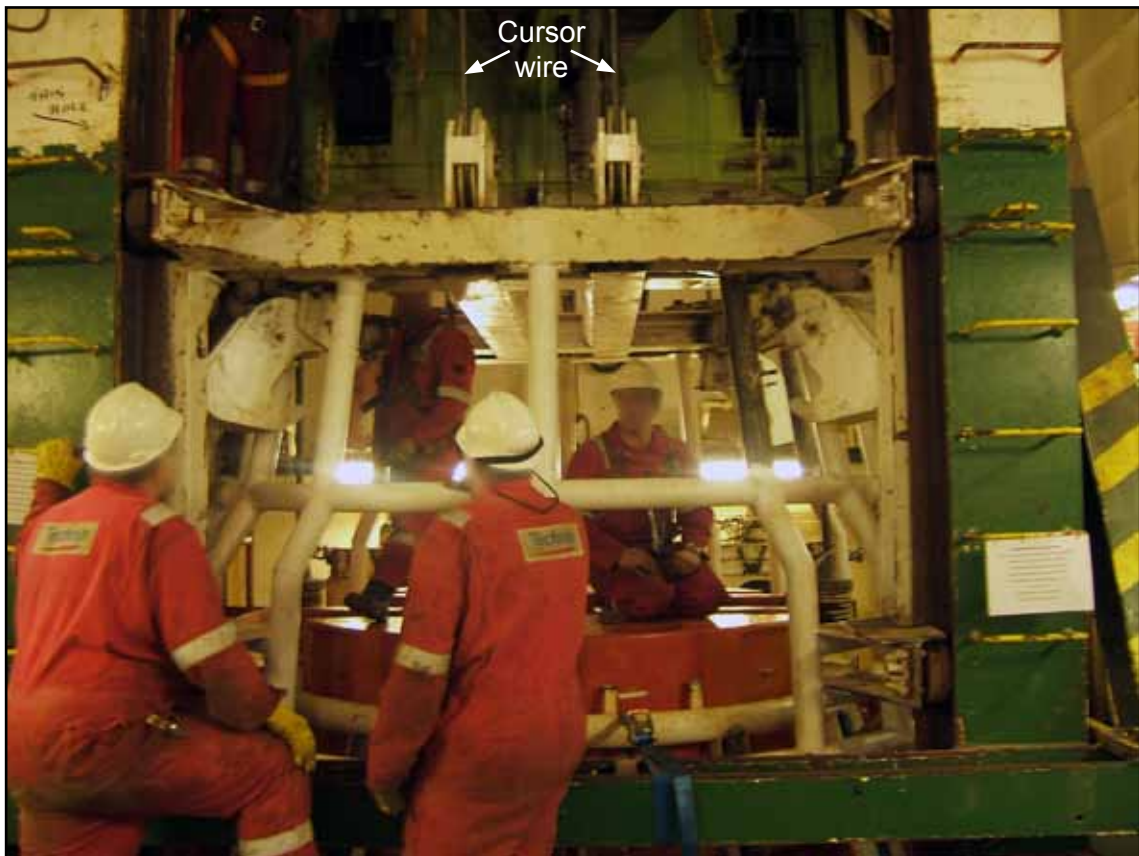
Riggers on top of the bell, under suspended cursor
