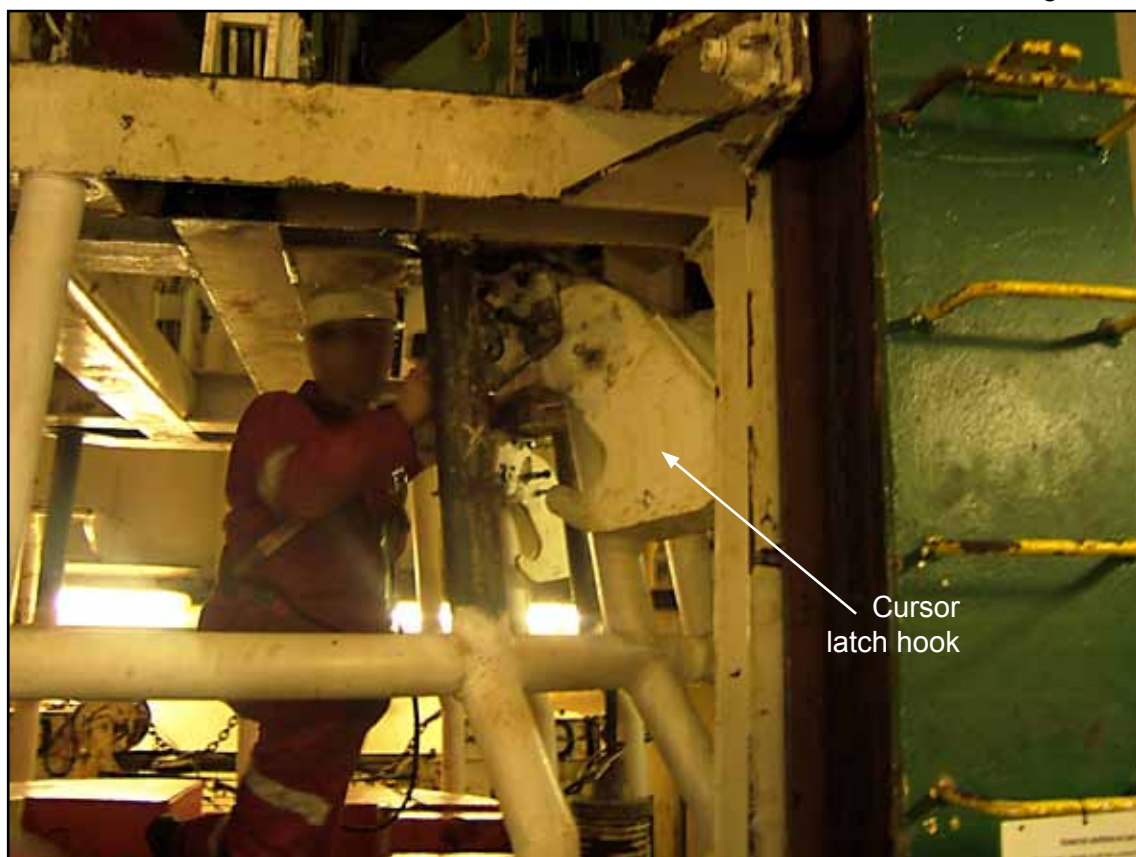
Rigger working on cursor latch hooks under suspended cursor
