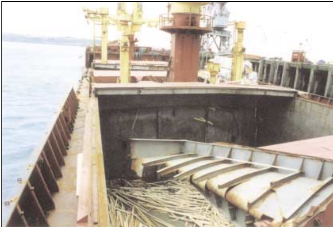
Photograph showing the damage to No 4 hold hatch cover
