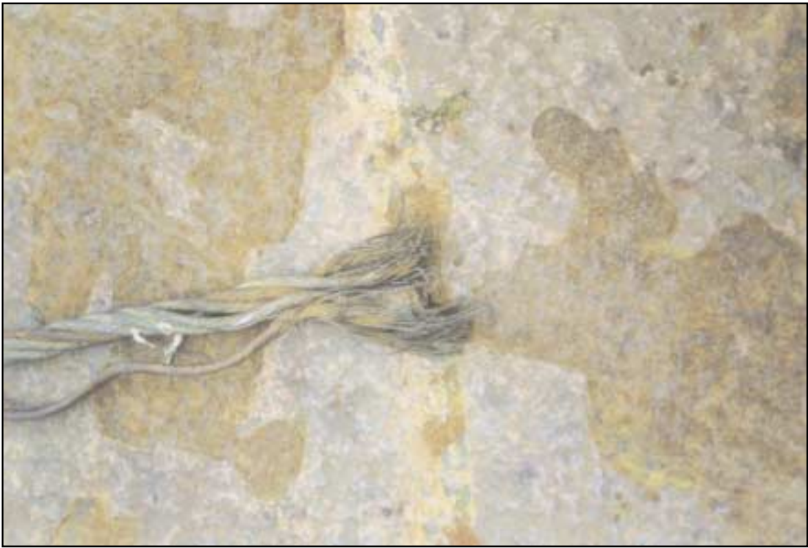
Photograph of stranded wire lashing
