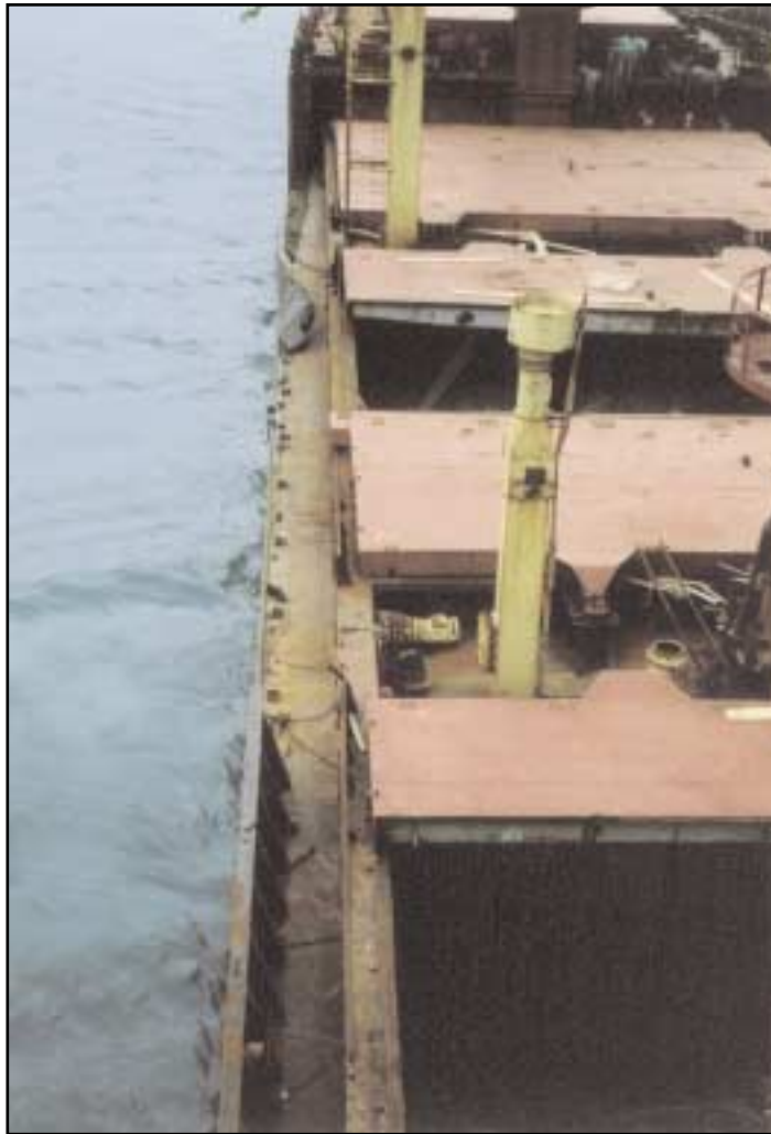
Photograph showing hold air vents
