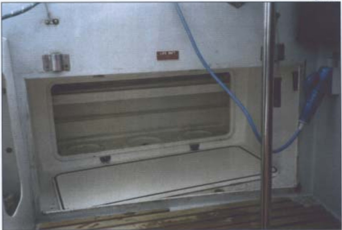
Spare gas bottle locker (one of two)
