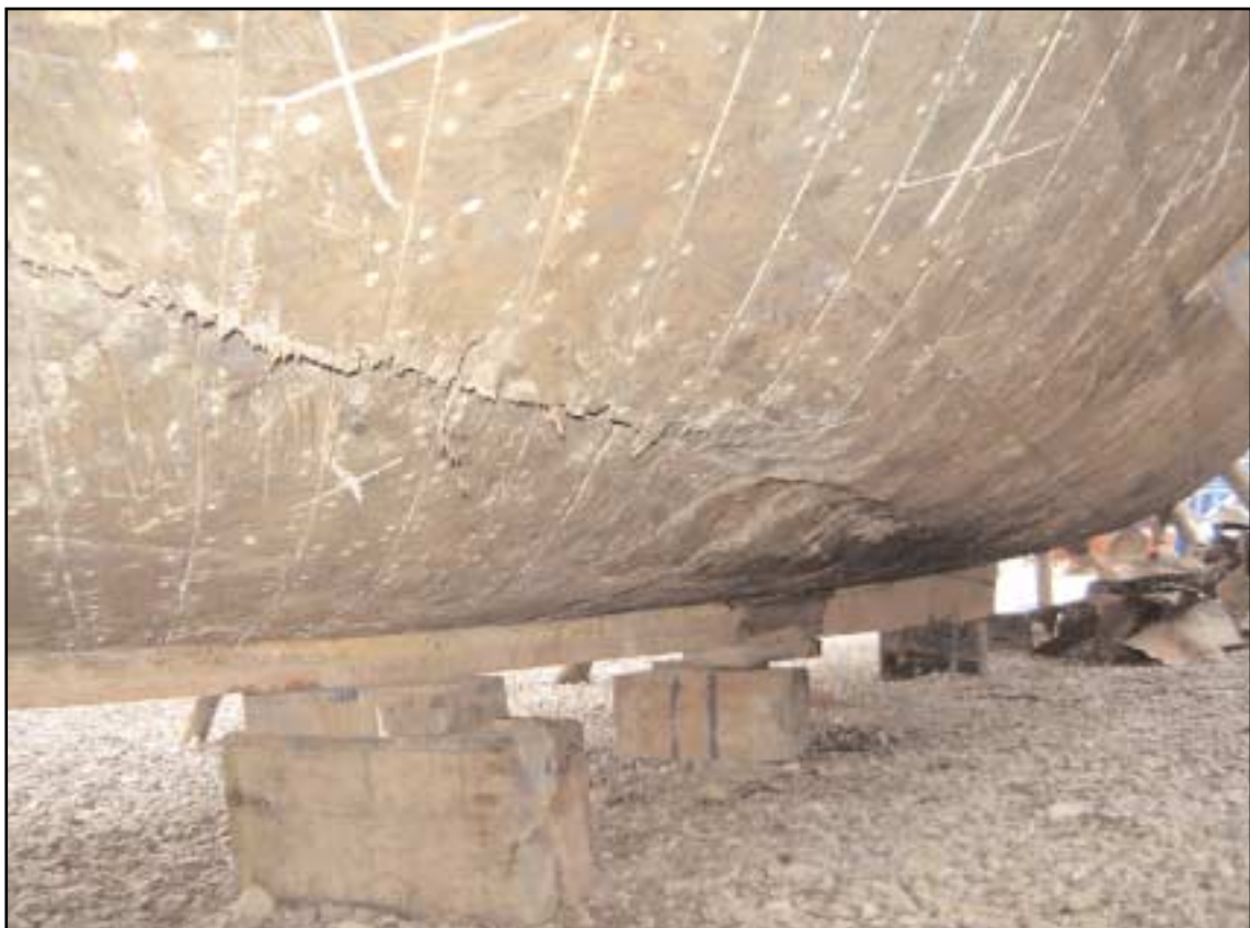
A view of the damage of the port side looking aft showing a longitudinal tear
