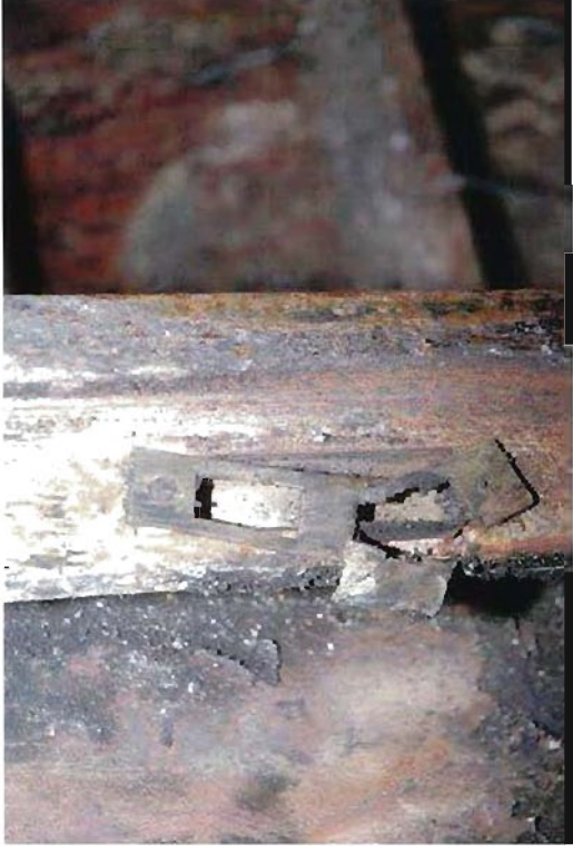
Photograph 39 The damage to the striker plate for the door to the Engine Store
