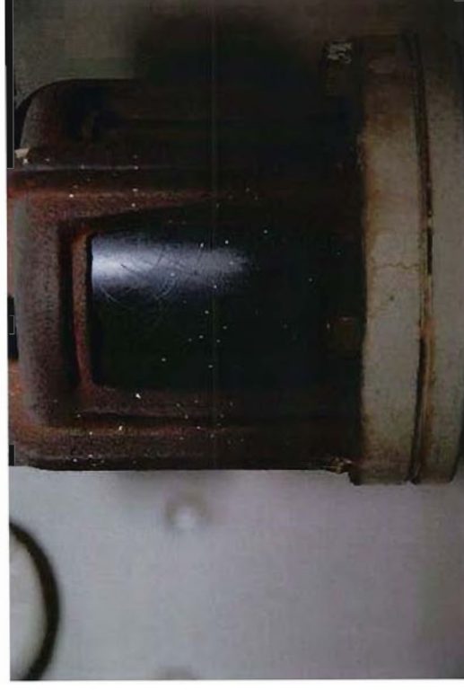
Photograph 35 The plastic sight glass in the Heavy FOT fuel line
