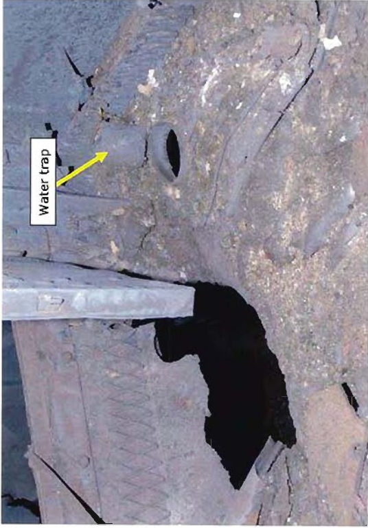
Photograph 37 The water trap for the Laundry drain in the fire debris.
